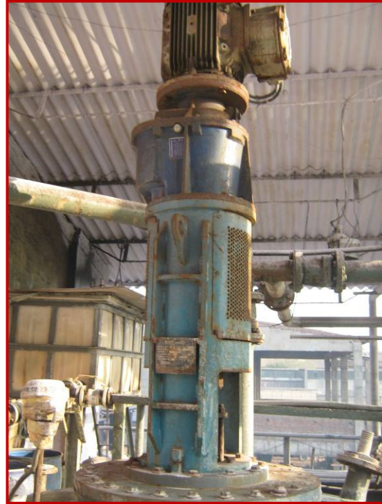
Figure 3.5: Operation of vertical agitator system at typical chemical unit
