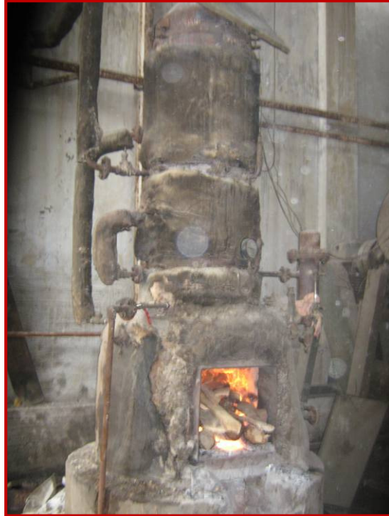
Figure 3.16: Operation of conventional wood fired Boiler at typical chemical unit
