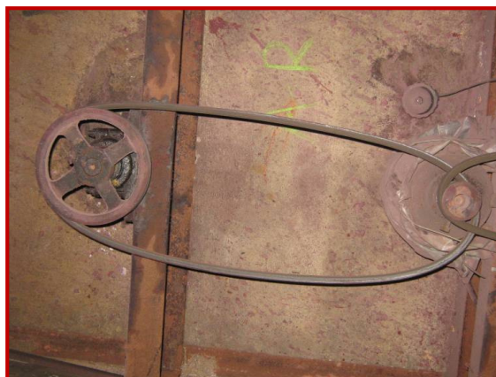
Figure 3.2: Operation of V-belts drives in typical chemical industry in Ahmedabad Chemical cluster
