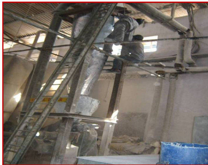
Figure 3.15: Insulation on cyclone chamber in spray dryer
