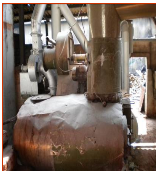
Figure 3.10: Energy efficient wood fired hot air generator at typical chemical industry
