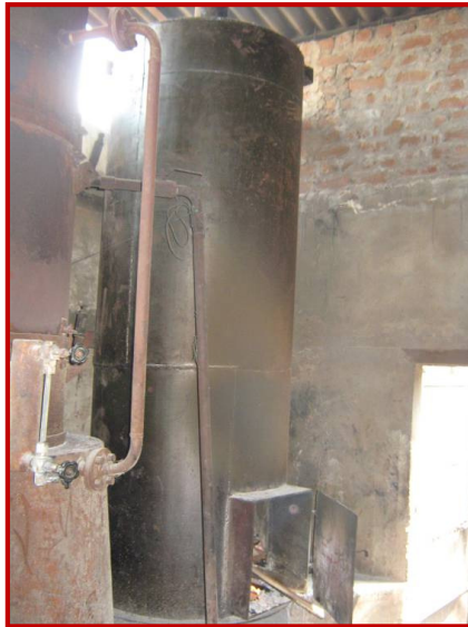
Figure 3.9: Operation of hot air generator without insulation over it
